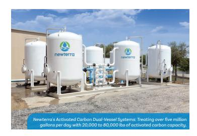
racks allow the dual-vessel systems to run in parallel or lead-lag. Pipe rack systems can include pressure relief valves, pressure gauges to monitor each vessel, and sample valves.
