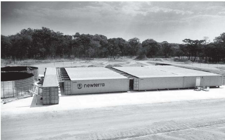
**MBR Wastewater System is Housed in 27 High Cube Shipping Containers Comprised of Distinct 3-Container Treatment Trains.**
